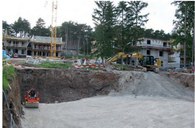
Fig. 9: GESIBA residential buildings (6) and (8) under construction; the construction pit for residential building (7) in the foreground. Photo: Christian Schubböck
