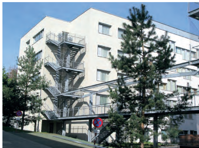
Fig. 10: VAMED building. Photo: Christian Schubböck
