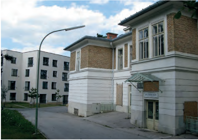
Fig. 6: The decommissioned pathology building and a new GESIBA residential building (4). Photo: Christian Schubböck
